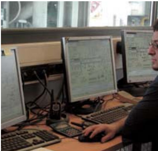
Scada Control System
