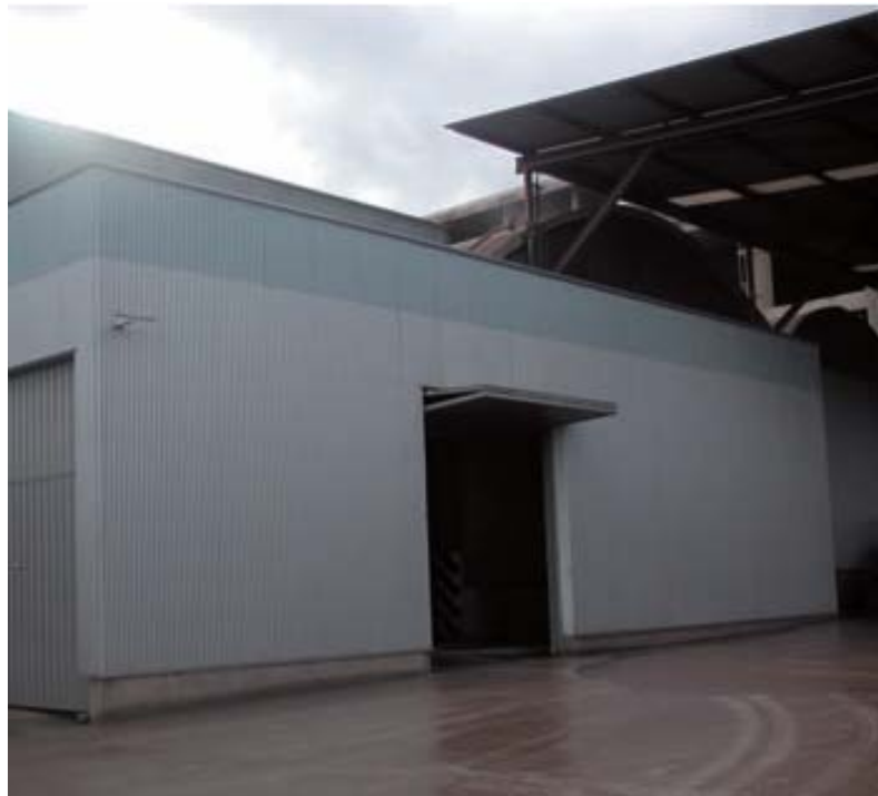
Lorry loading shed
